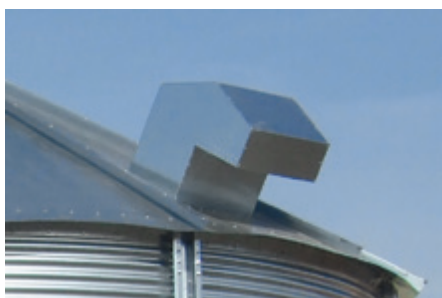
ROOF VENT – allows to remove moisture from the ventilated grain
